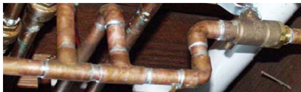
Even though the use of lead solder was banned in the U.S. by 1986, it still might be present in older homes.
